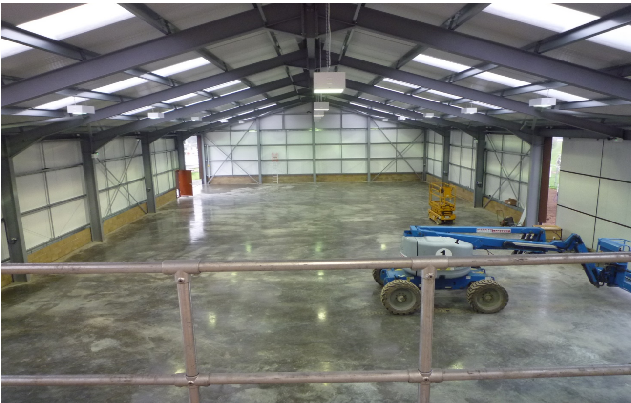
Photo taken just before completion
